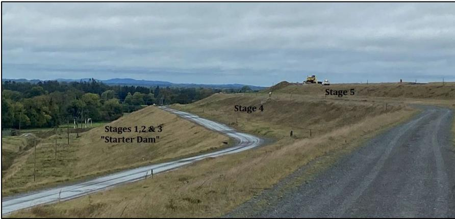
Figure 6.2: Embankments side profile
